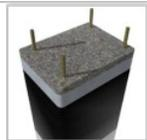
**Column strengthening by means of CFRP confinement.**
