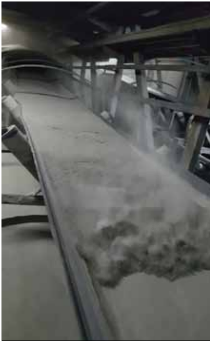
Figure 2: backflow of cement on an inclined conveyor belt due to high powder flow
