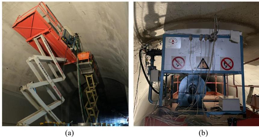
Figure 1. (a) Application of Sikacrete<sup>®</sup>-213 F to the tunnel crown and (b) furnace for site fire resistance testing in the Panagopoula twin railway Tunnel.
