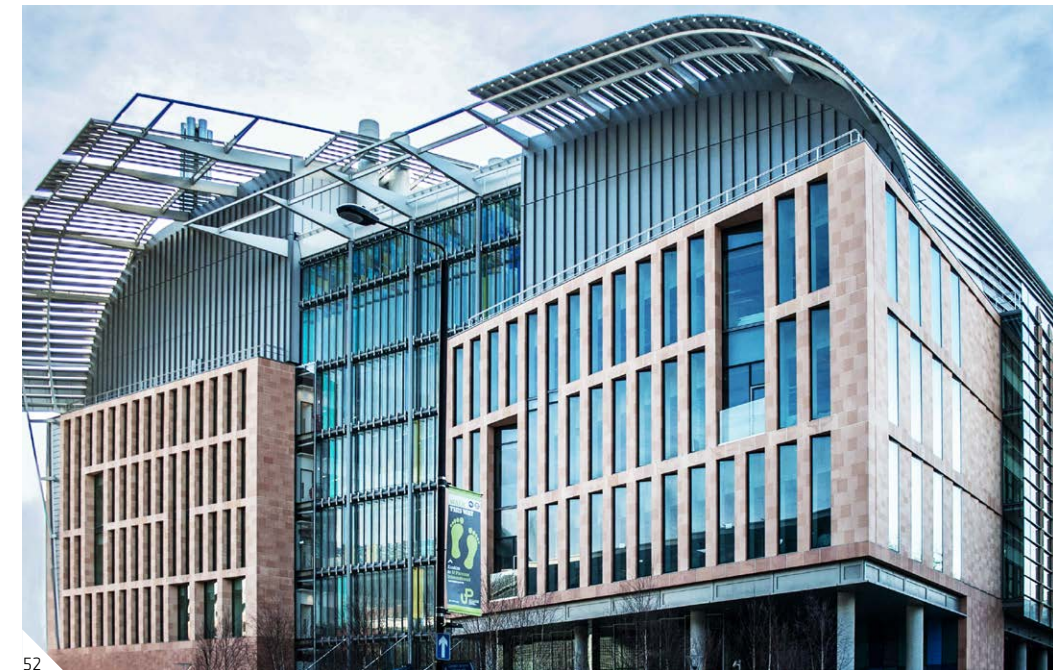
Francis Crick Institute Project Participants Architect: HOK, PLP Architecture Facade: Scheldebouw, Josef Gartner (2016)
