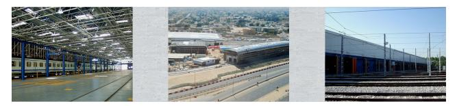
Any METRO systems need a Depot where rolling stock will be stored, maintain or even repaired. Usually located above ground, they consist of large hangar where different and specifc facilities will take place. These structure are usually made of concrete and steel.
