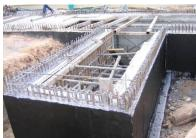
WATERPROOFING LININGSikaProof® Membrane, SikaTop® Seal 107SikaProof® MembraneBitumen modified elastic liquid applied membraneSikaTop® Seal 107Flexible Protective and Waterproofing Slurry. 2 compo-<br/>nents mortar for basement, wet area, drinking water<br/>tank. Sikagard® range Epoxy base protective coating<br/>for steel or concrete
