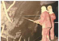
**DEWATERING** SikaShot® SikaShot® Ready to use waterproofing gunite with very fast setting to seal water seepage by spraying
