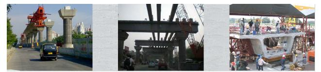
Elevated systems are built as Viaduct construction, where large parts of the structure require typically Reinforced Concrete structures.
