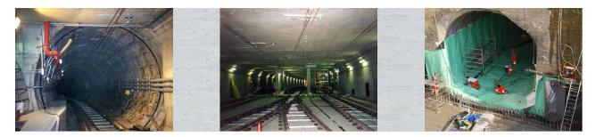
The use of TBM-technology is the most common excavation method due to the local geology and hydrology. Once built, the tunnel system shall guarantee a safe and a dry environment for any Metro users. Optimized cost and easy maintenance will be the key objectives for any solutions.
