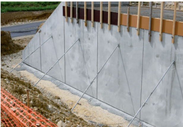
Precast concrete elements
