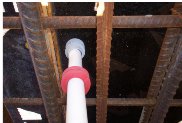
Formwork spacers
