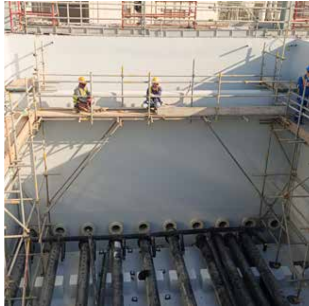
Desalinated potable water storage tank, Al Khobar, Saudi Arabia: 90,000 m 2 of Sikafloor®-161, Sikagard® PW.
