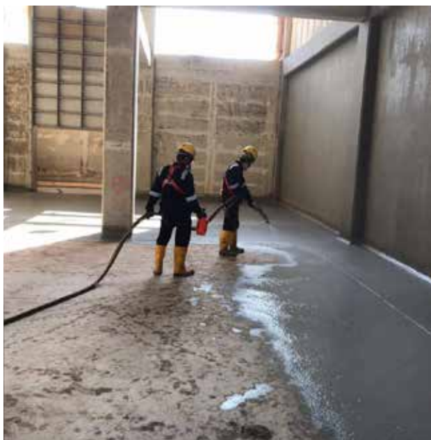
Rapid refinery Pengerang, Malaysia: Tank refurbishment with Sikalastic®-1K (spray application), Sikadur® Combiflex® SG Tapes and Sikaflex® PRO-3.
