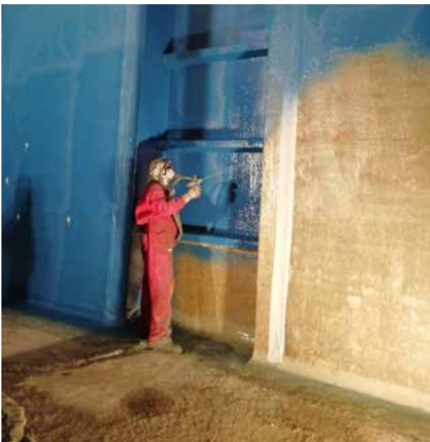
Reservoir Santa Cruz del Valle, Spain: 1,800 m 2 of Sikafloor®-161, Sikalastic®-840 ES.
