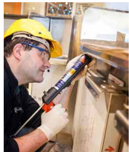
Fig. 9 Application of Sikaflex®-291i
