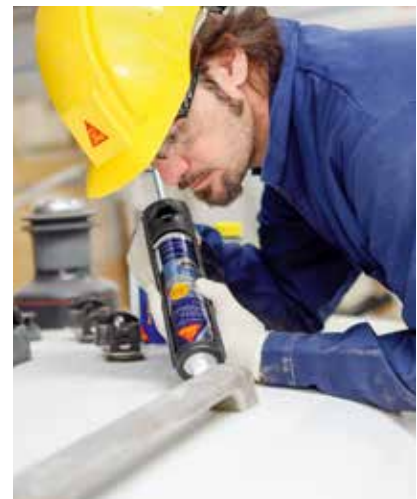
Fig. 5 Sealing the edge of a chrome hand-rail
