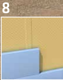
8 WT protection sheet/ felt and thermal insulation boards
