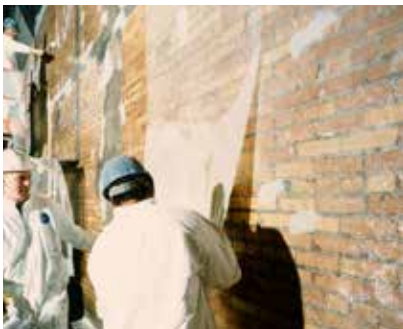
SEISMIC UPGRADING /EARTHQUAKE DAMAGE REPAIR
