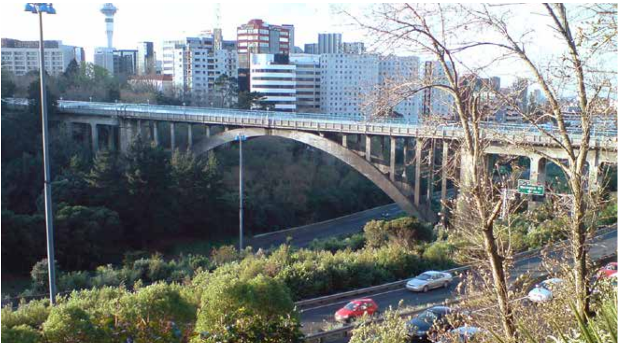
Grafton Bridge, Auckland, New Zealand
