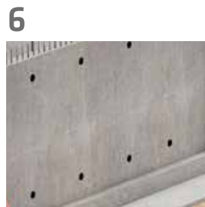
SikaSwell® Rings and Plugs Sikadur® 31 Sealing tie bar holes
