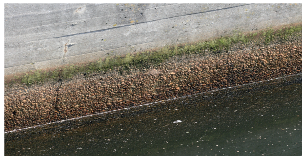
Heavy leaching and damage to the structural concrete are observed particularly in the water splash zone of biological treatment basins.
