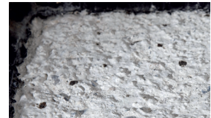
Very severe surface weathering
