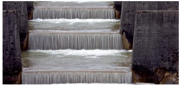
Particularly in whitewater, concrete surfaces are subject to massive additional strains by rubble, sharp edges and abrasion, as well as possible temperature stresses due to frost exposure.
