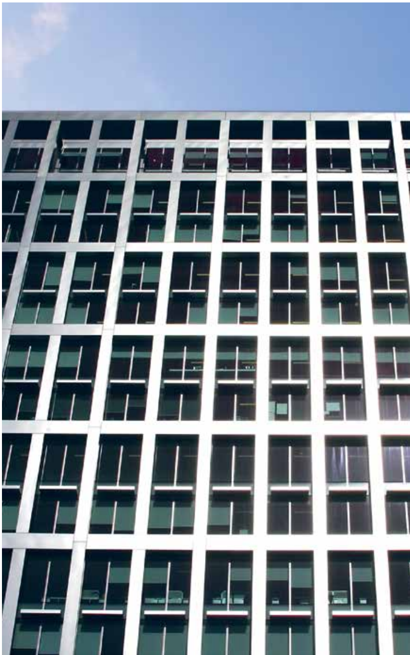
top left: 5 Aldermanbury Square, London, 2005 Architect Eric Parry Architects; Facade Lindner-Schmidlin UK
