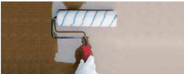
Primer application with a medium pile roller.
