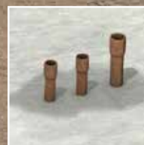
Leaking Penetrations i.e. Pipe Penetrations
