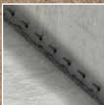
Leaking Construction Joints
