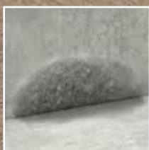
Leaking Areas of Voids i.e. Honeycombing
