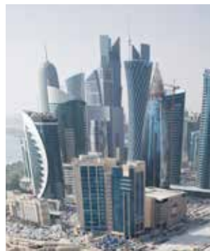
COMMERCIAL OFFICE BUILDINGS
