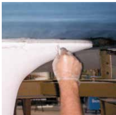
Fig. 13 The joint is tooled off and finished
