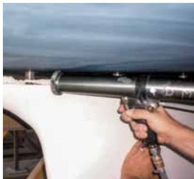
Fig. 12 The adhesive is applied
