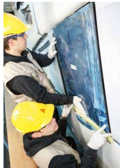
Fig. 7 The window is fitted
