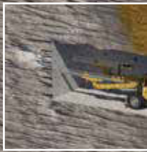
Control of over-blast
