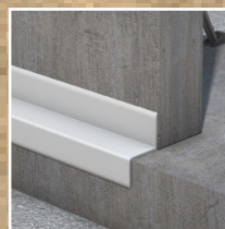
Connection joint between of precast elements
